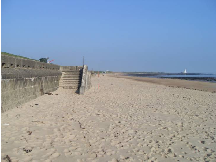
Plate 3 – Survey photograph 1aNTDC03_20120322_N2.JPG
