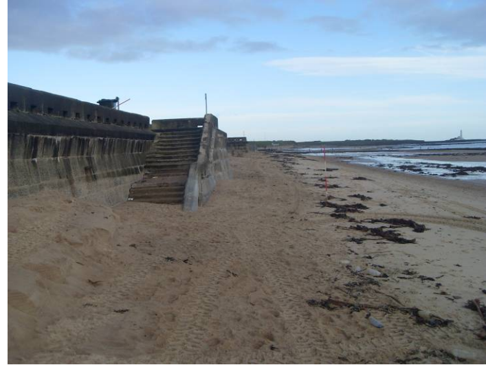
Plate 4 – Survey photograph 1aNTDC02_20120928_N2.JPG
