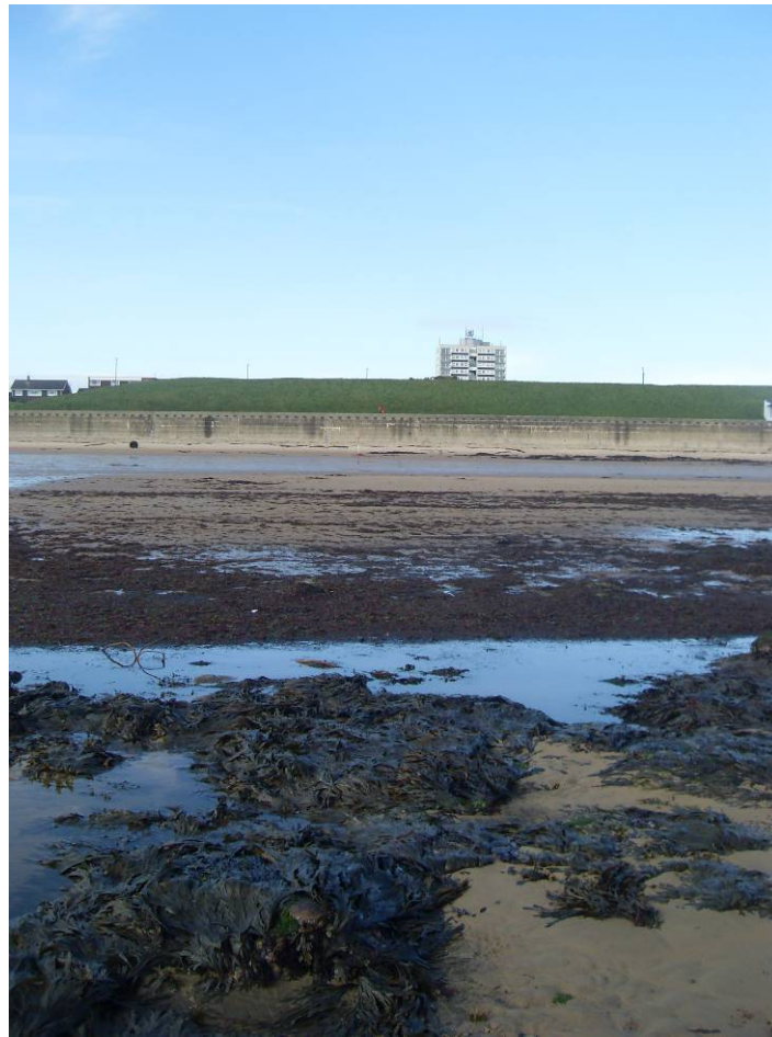
Plate 2 – Survey photograph 1aNTDC02_20120928_Up2.JPG
