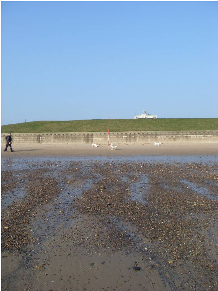
Plate 1 – Survey photograph 1aNTDC02_20120322_Up1.JPG
